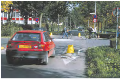
Culemborg junction: Traffic signals removed and entrances narrowed.
