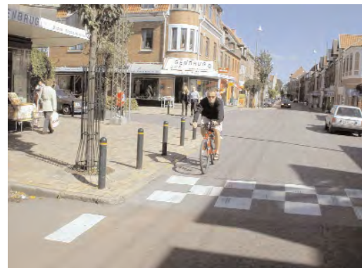
Odense: Conventional road markings removed.
